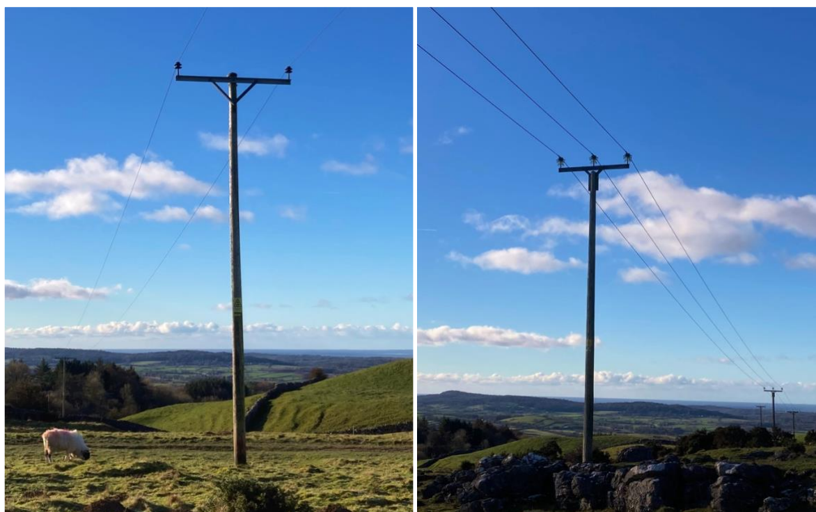
Figure 10: Left: a single-phase power line. Right: a three-phase power line
