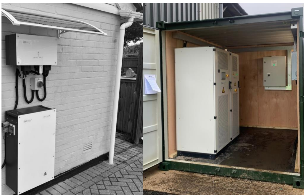
Figure 19: Real examples of domestic (left) and commercial (right) battery locations
