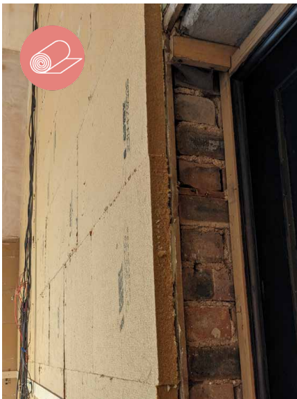
40mm breathable wood-fibre insulation panels are installed to all internal walls, co-ordinated around architectural features
