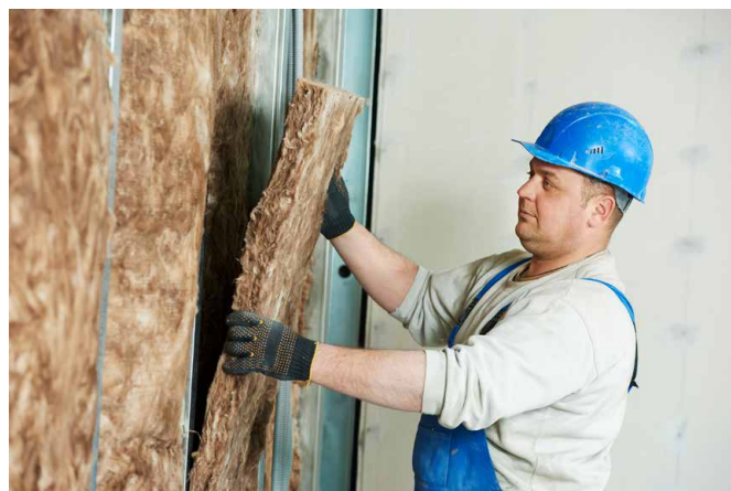
Internal wall insulation
