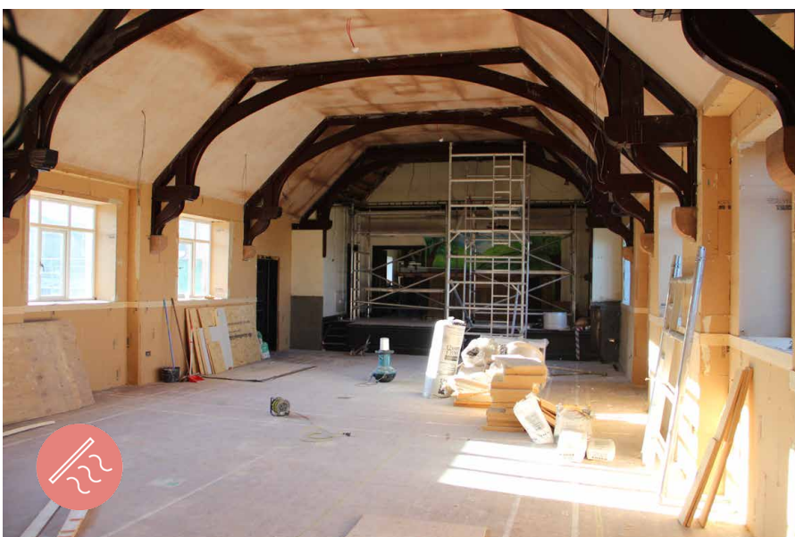
The main hall space with walls insulated and ceiling recently plastered
