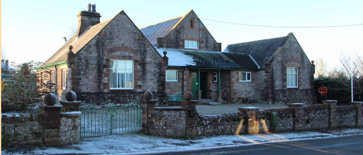
Skelton Toppin Memorial Hall, 2023, with solar PV panels now just visible on the central roof
