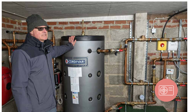
The internal part of the ground source heat pump is located in a semi-basement beneath the stage area
