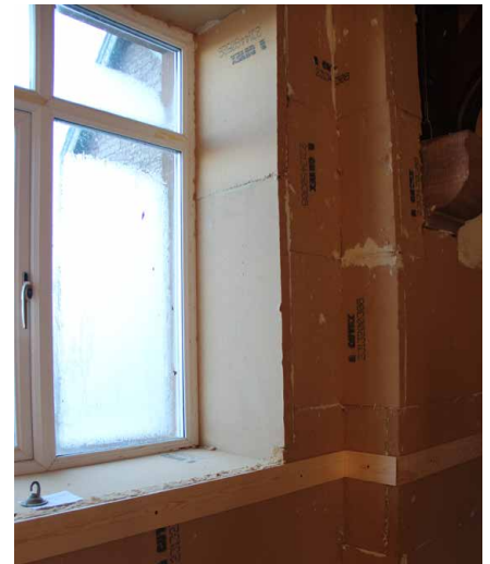
Wood-fibre board insulation fixed internally and turned into the reveals to meet the window frame at Skelton Toppin Memorial Hall.
