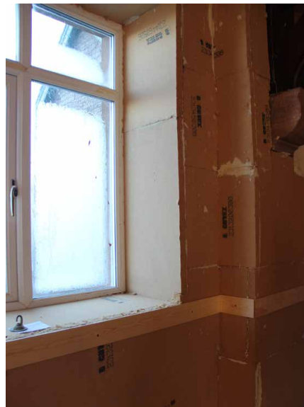
40mm breathable wood-fibre insulation panels are installed to all internal walls, co-ordinated around architectural features
